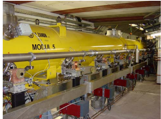
Fig.4: Module ACC 5 equipped with the TTF 3 couplers. Above the couplers the common pumping line for all 8 couplers is seen. Below the couplers the wave guide distribution system with the remote controlled three stub wave guide tuners, directional couplers and circulators is assembled.
