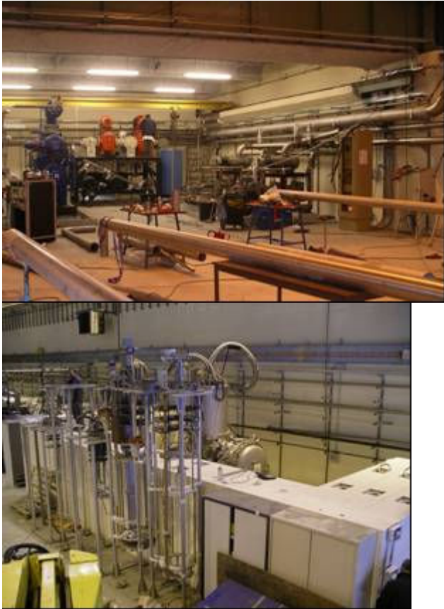
Figure 10.6. Re-installation of the helium compressor and vacuum pumping system (left) and the CryHoLab area (right).
