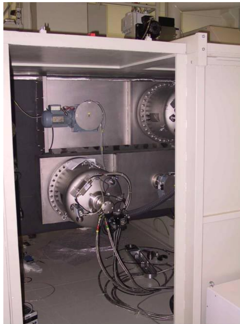
Picture 3: Cryogenic pumping station with 20.000 l/s
